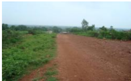
View of approach road to the site
